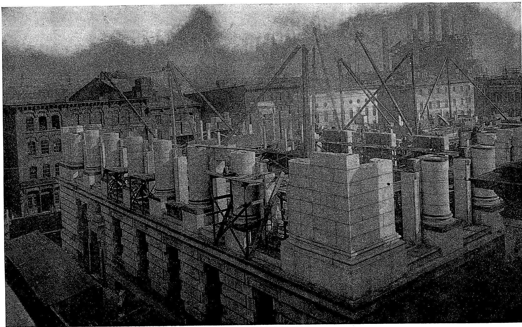
Customs Building, Baltimore, Md., under construction. Built of Winnsboro Blue Granite.
