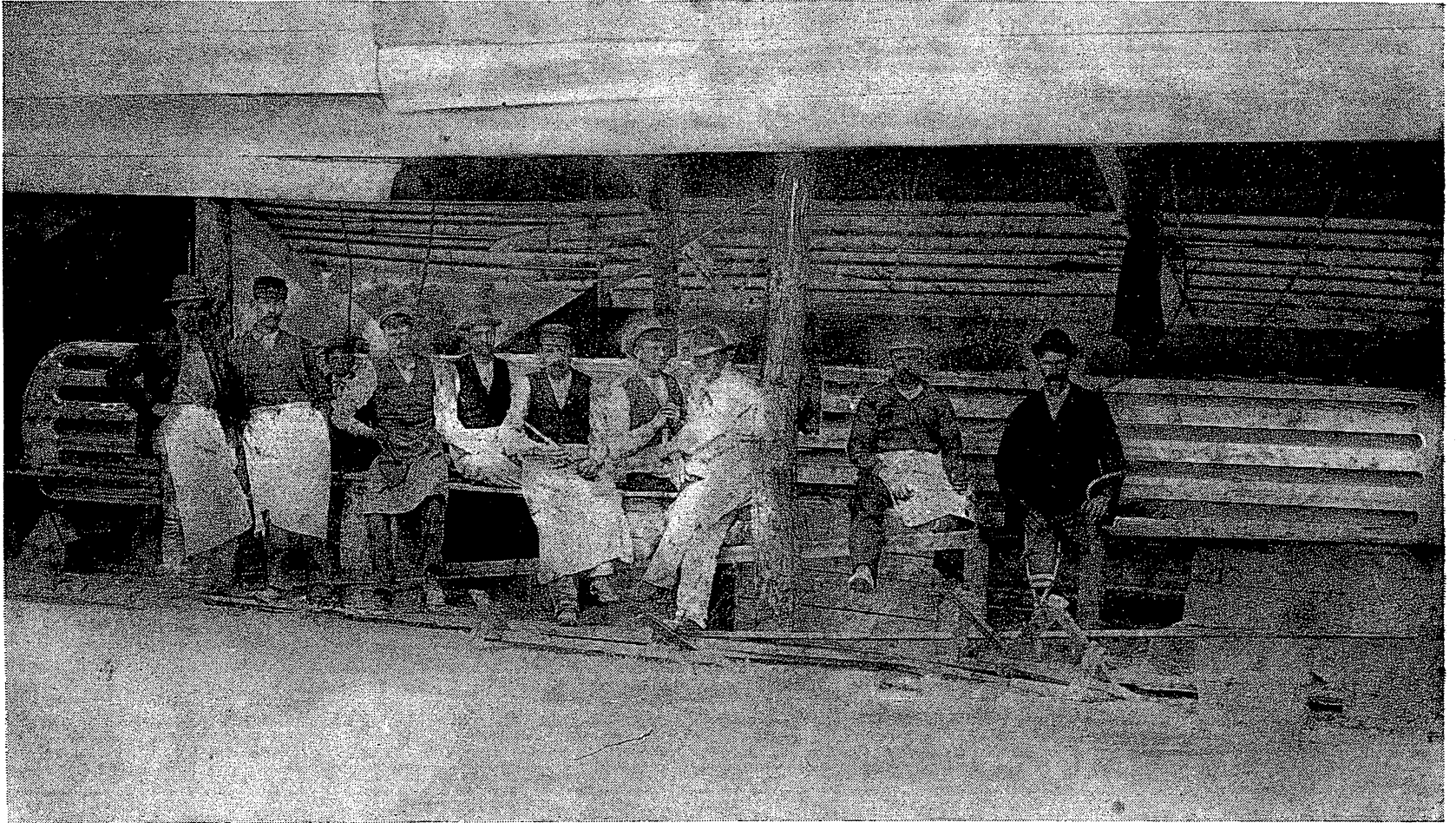
The stone column shown in the above picture is thirty feet and one inch long and four feet, two and a half inches in diameter. The men in the picture have just completed cutting this large column out of Winnsboro Granite at Rion, S. C., for use in the construction of the Land Title & Trust Building of Philadelphia, Pa.
